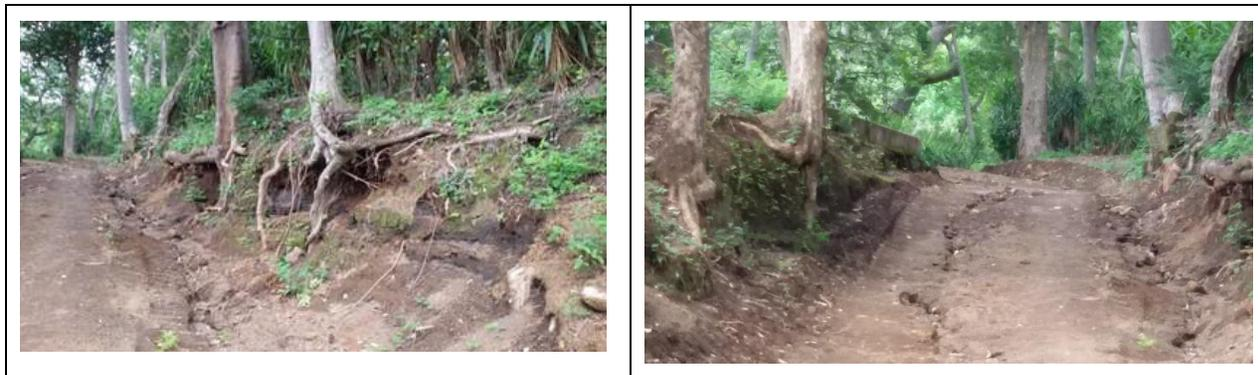
Figura 14: Taludes inestables del camino
